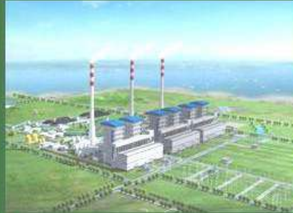
3960 MW Mundra, Adani Power Ltd
